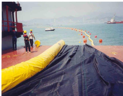
Figure 9 - Photograph of deployment of the Silt Screen on a previous project
